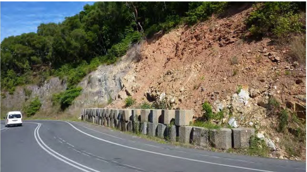
Recent Cutting Instability and Old Linemarking Evident
