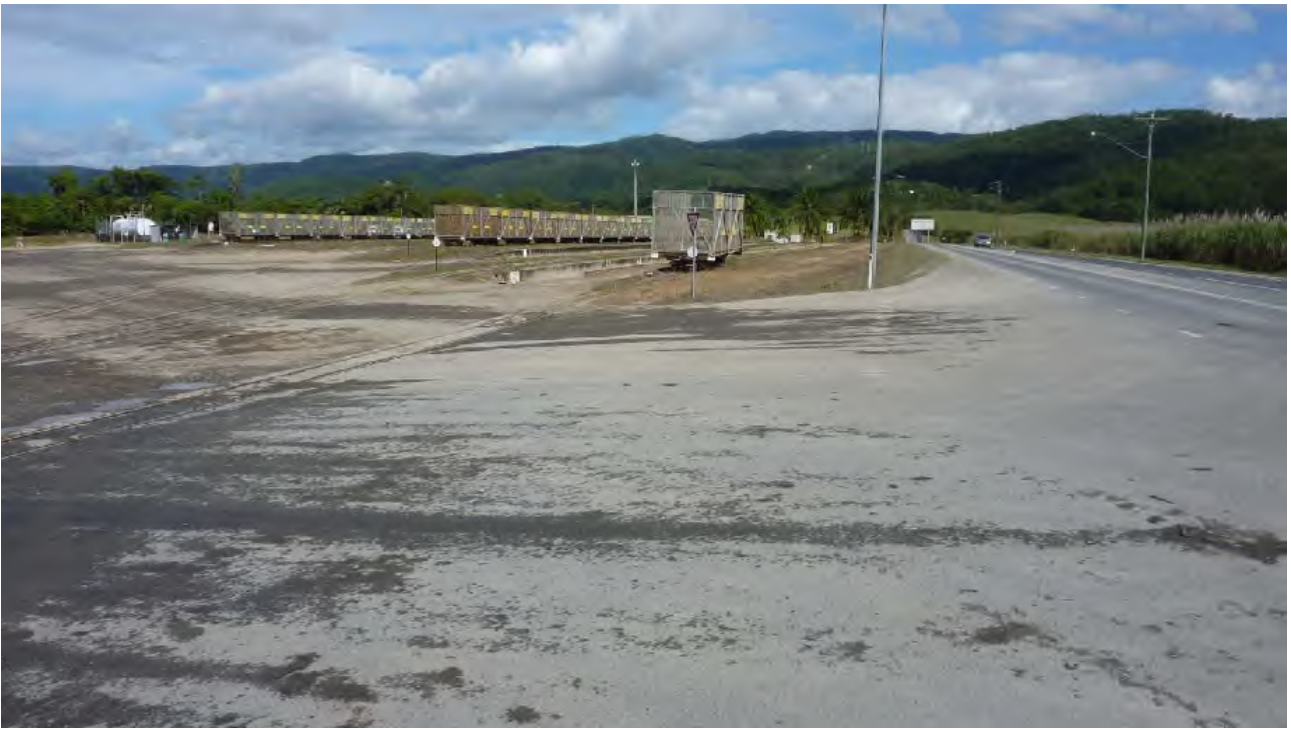
Mud & Dirt Obscuring Road Pavement Markings
