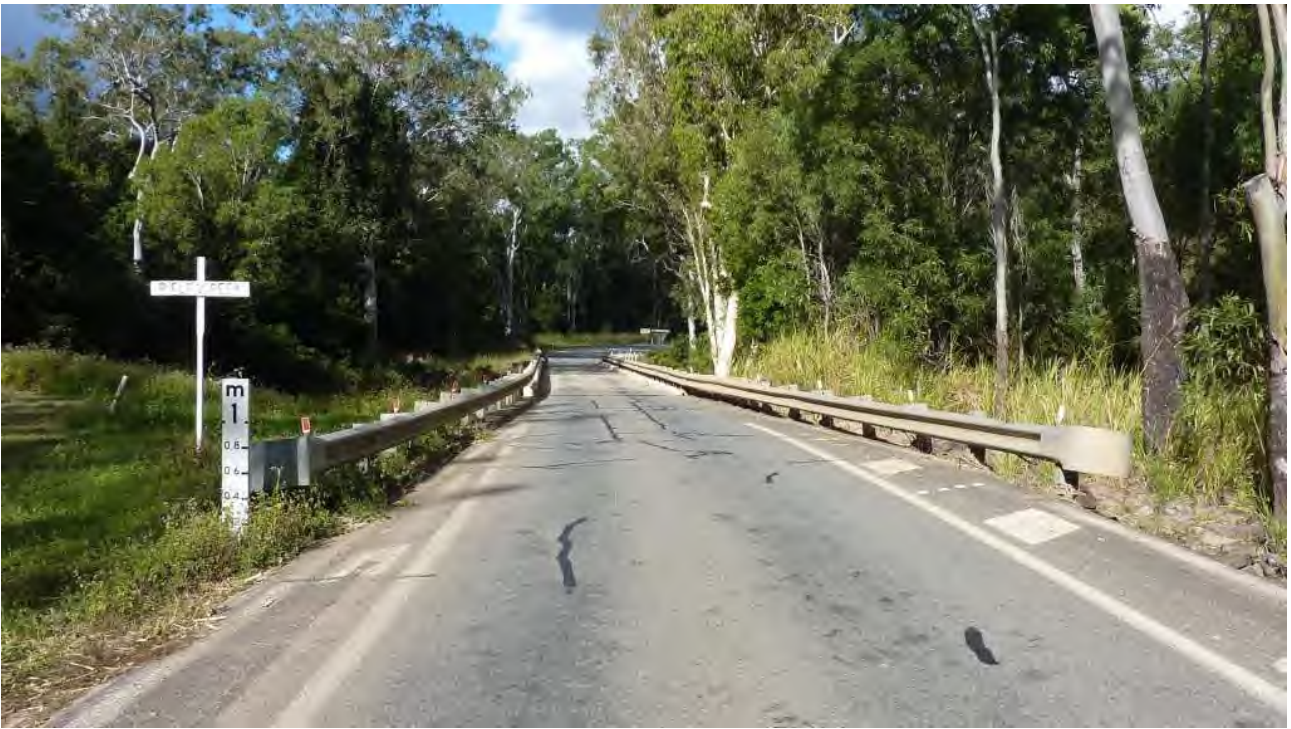
Delineation – Terminal End Treatments Missing
