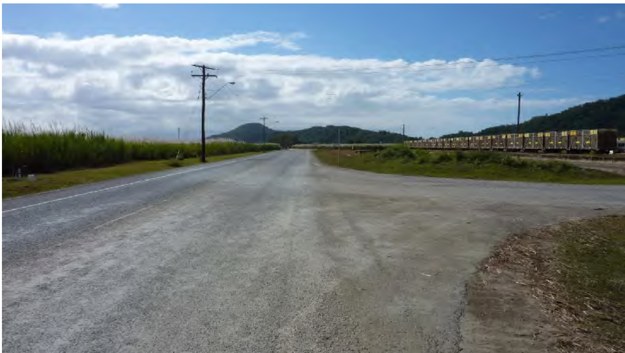
Entrance to Cassowary Siding for HV – Minimal Intersection Treatments for turning Vehicles
