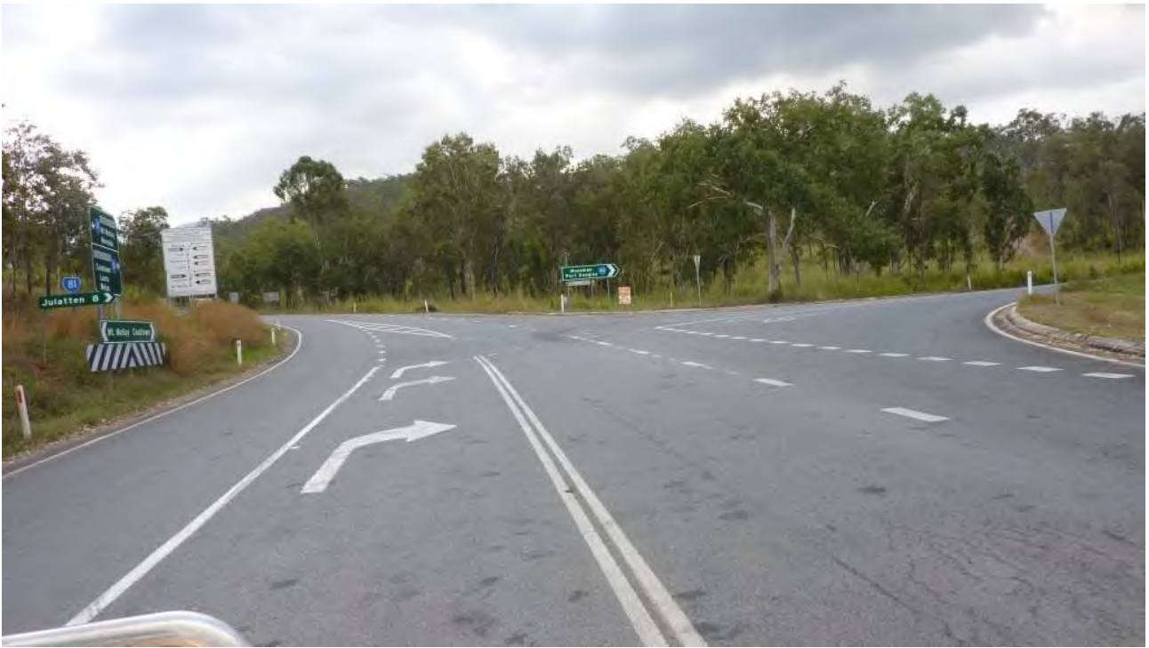
Restricted Sight Distance for RH Turning HV
