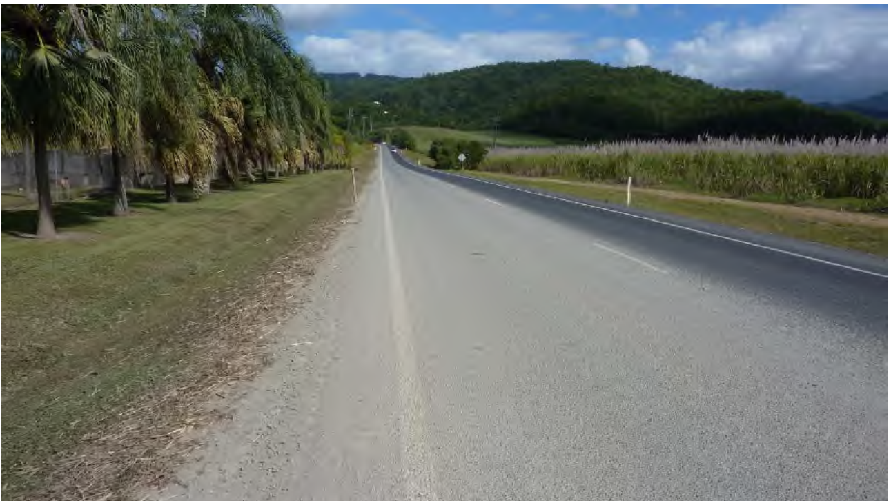
Pavement marking obscured
