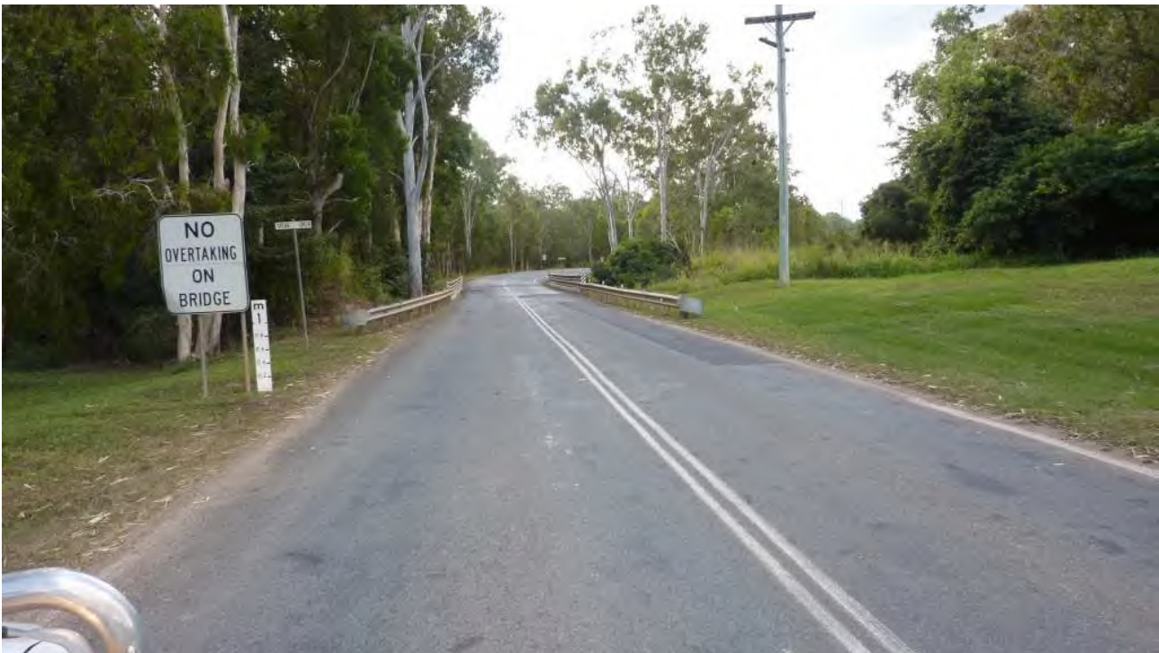
Delineation – Terminal End Delineation Missing
