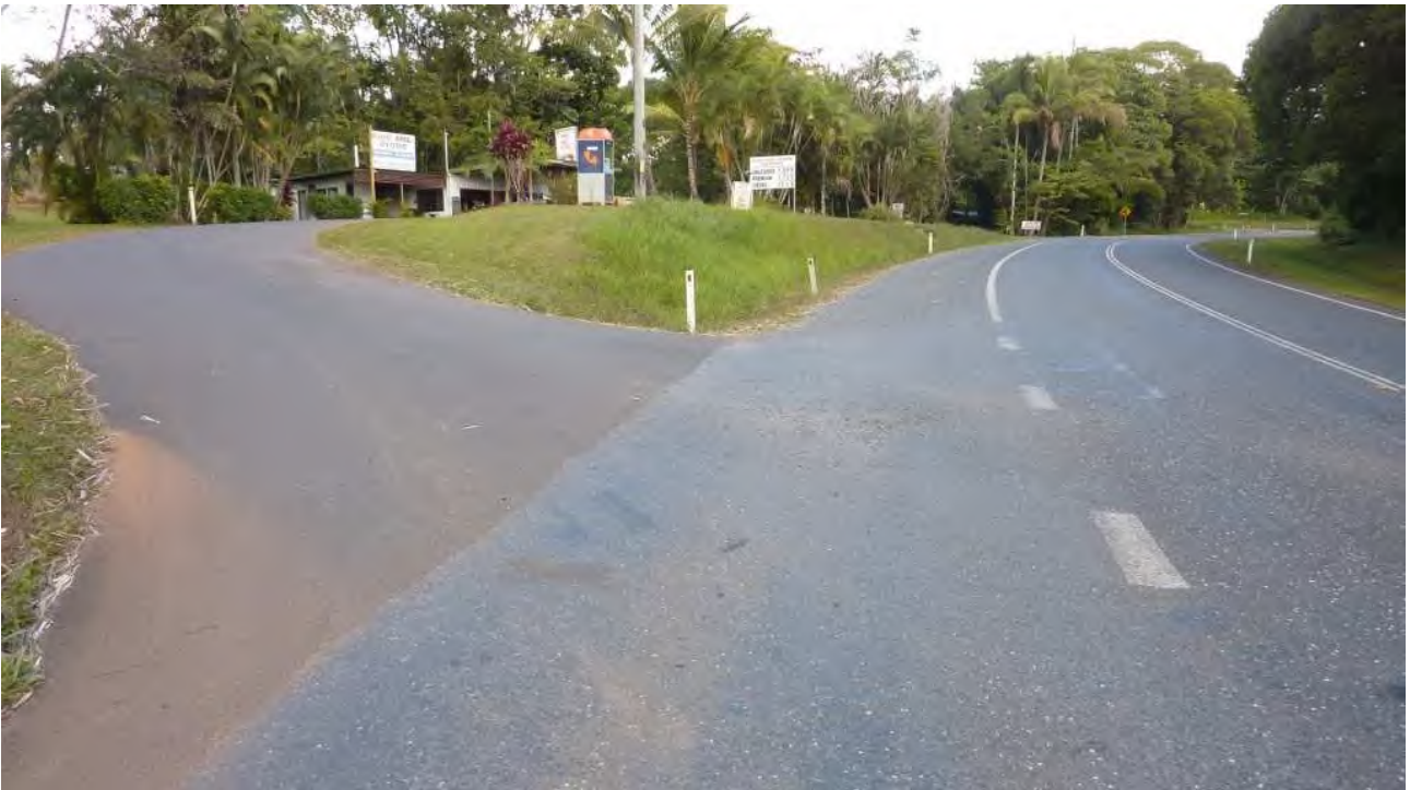
Adjoining impervious areas and discharge of concentrated sheet flow to carriageway on curve
