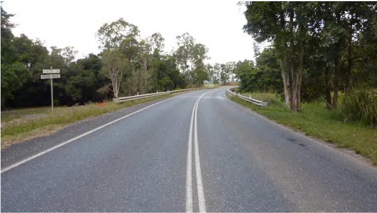
Delineation – Terminal End Delineation Missing
