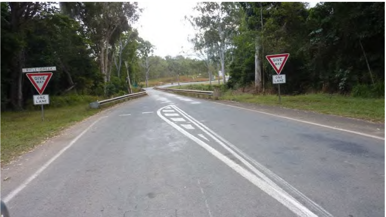
Delineation – Terminal End Delineation Missing
