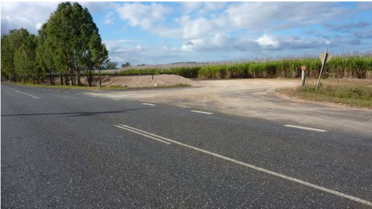
Access to Cane Bin - Loose material on roadway
